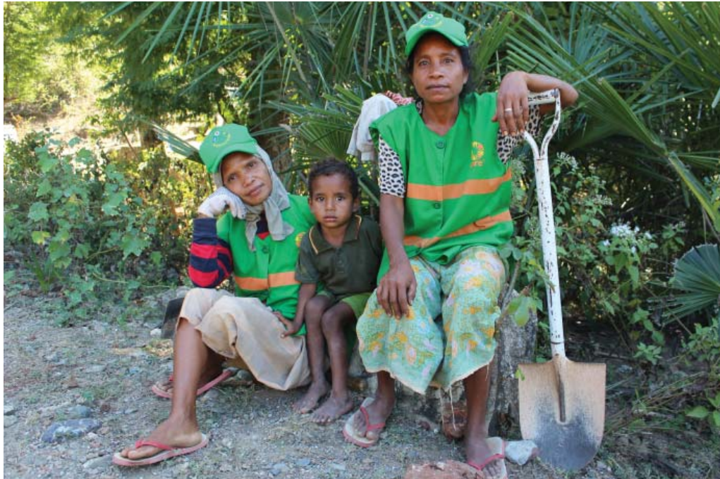
Women community road maintenance workers in Maliana (Bobonaro District)
